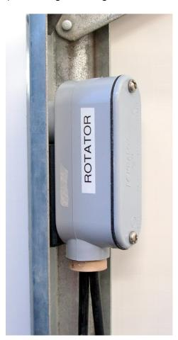
This allows you to easily disconnect your inside rotator control box, and substitute another rotator control box outside, where you can see the antenna, and communicate with the guy up on the tower.
